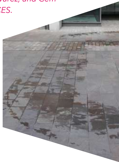
Figure 1. Water traces left by ride-on sweeper after cleaning shift, The Canopy , King's Cross (autumn 2017). Photo: Adriana Cobo
